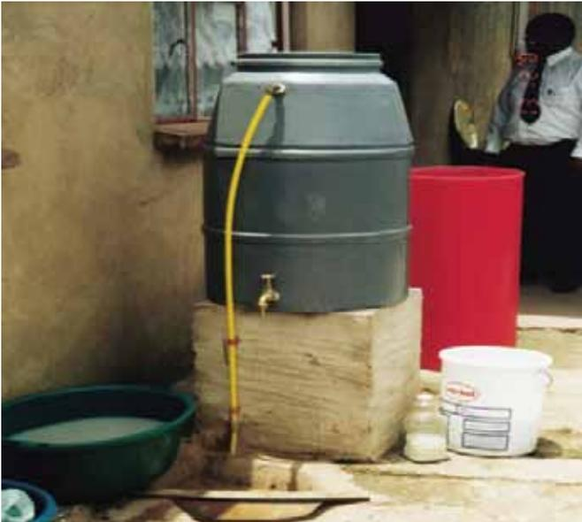
*Low pressure (ground tank) with yard tap and associated drainage channel (soak away).*
